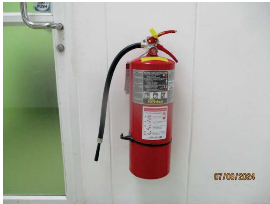
Portable Dry Chemical Extinguisher
