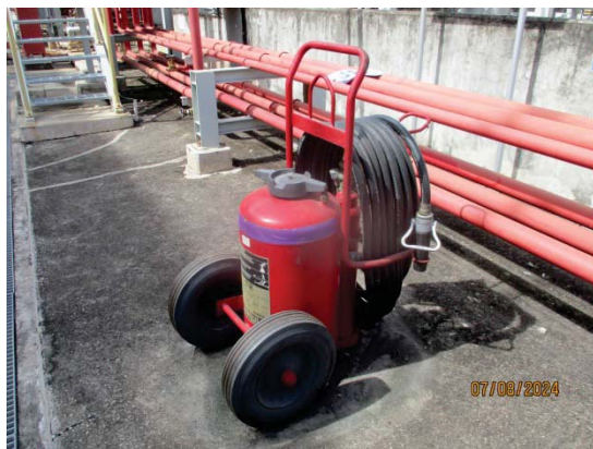
Wheel Dry Chemical Extinguisher
