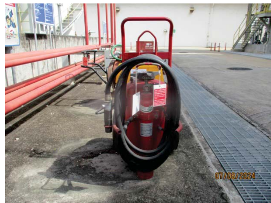
Wheel Dry Chemical Extinguisher
