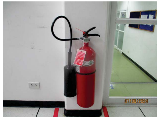
Portable Fire Extinguisher (CO 2 )
